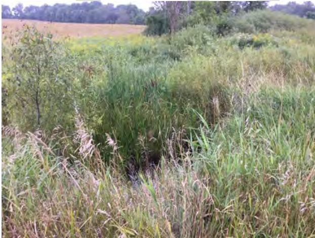
Crossing under County State Aid Highway No. 4 view of culvert.
