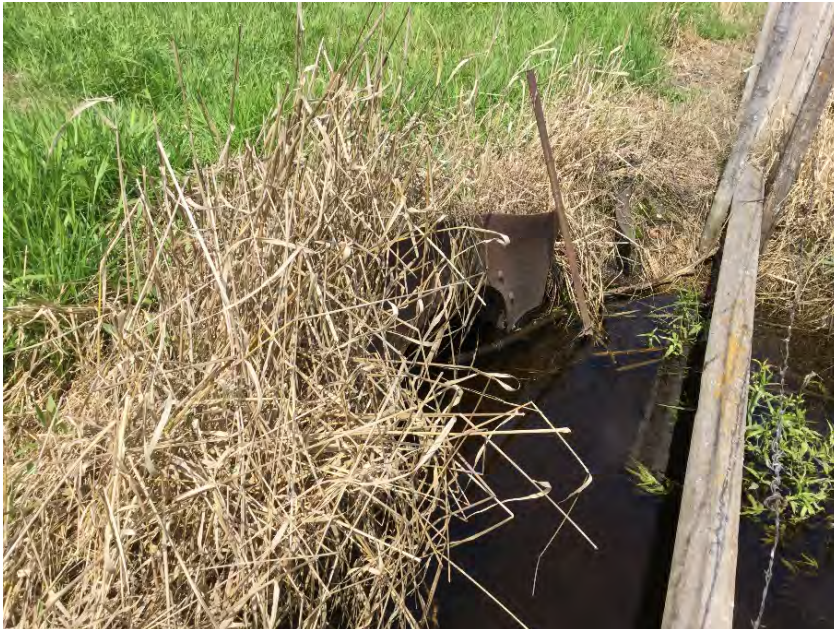
Private crossing east end culvert
