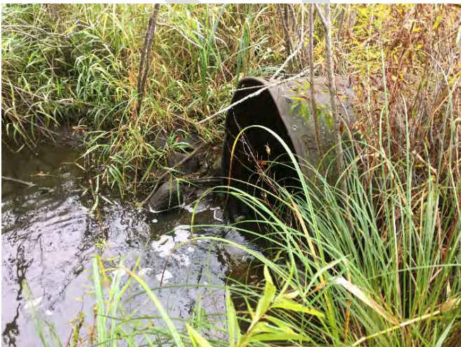
Private crossing west end of the culvert
